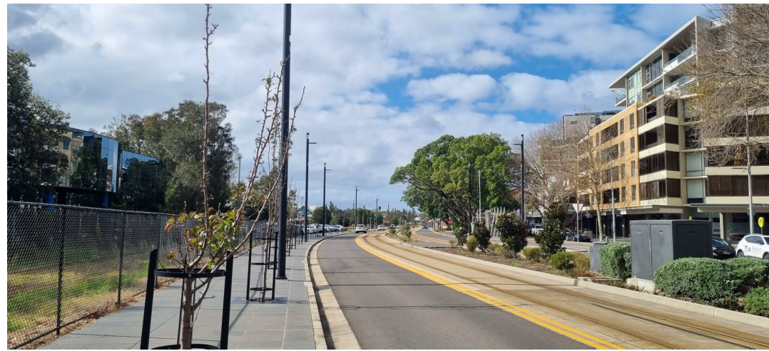
4 VIEW EAST DOWN HUNTER ST
