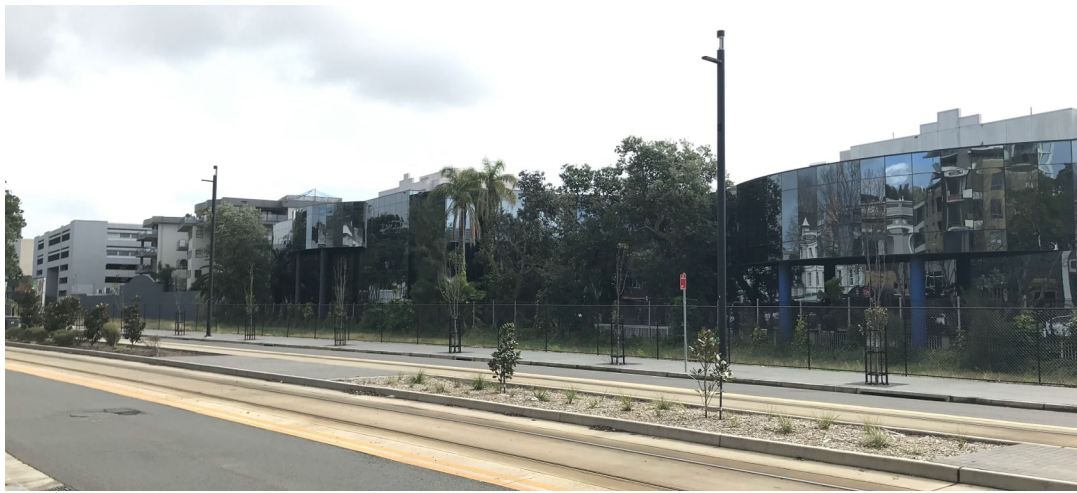
3 REAR OF BUILDINGS FROM HUNTER ST - FUTURE LANEWAY
